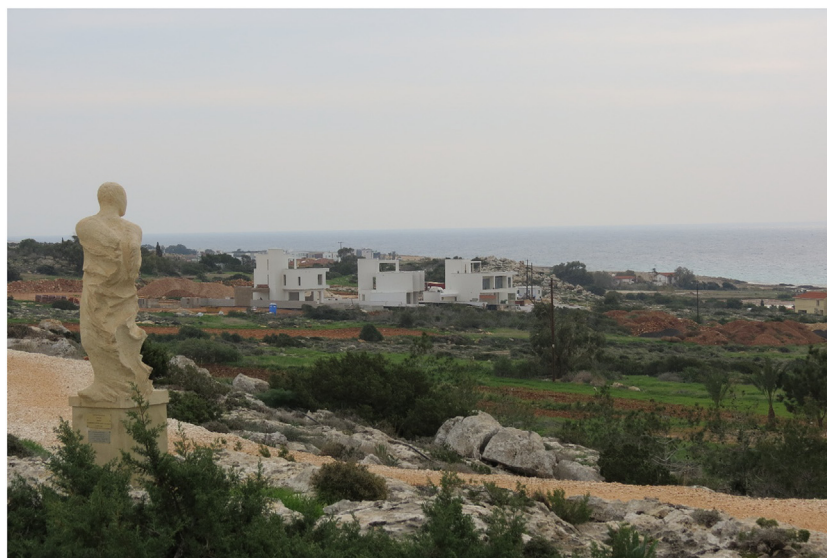
Photo 1. Holiday houses under construction in the distance.
